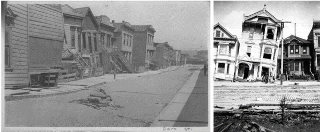
Figure 14.79 Photos Above Show Two Low Lying Areas in San Francisco After the 1906 Earthquake, Much Damage Was Contributed to Liquefaction. Image is in the public domain.
